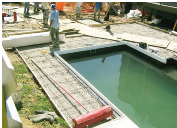
As Ryan Fisher builds his swimming pool and fence, no one seems to dispute the legality of his addition including city inspectors, but some residents, including Alice Gomez, questions whether this whole matter could have been handled in a more neighborly way.
